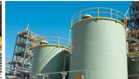
to the measure tanks in which the oil is separated from the rest of the liquid. The remaining water is then pumped from the measure tanks to holding tanks for treatment.
